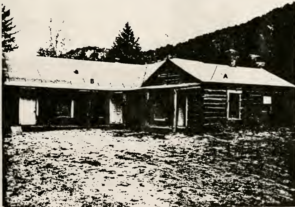
Figure 192. Structure #70, northeast view. A) original log building B) addition
